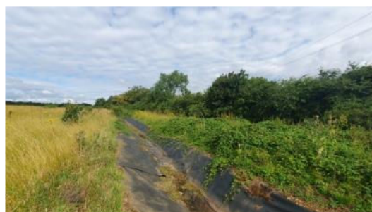
Photograph 12. Lined drainage ditch.
