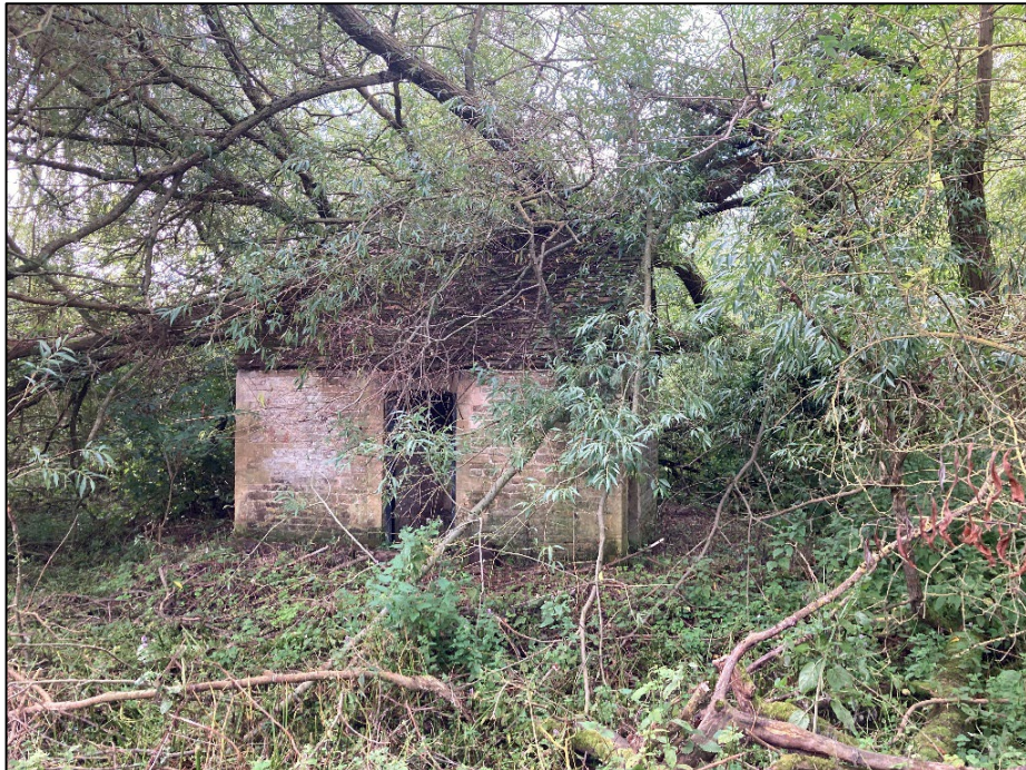
Figure 14 The lavatory block
