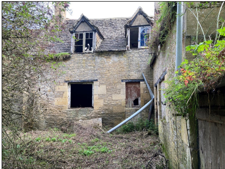
Figure 12 Centre of rear elevation from the south looking north
