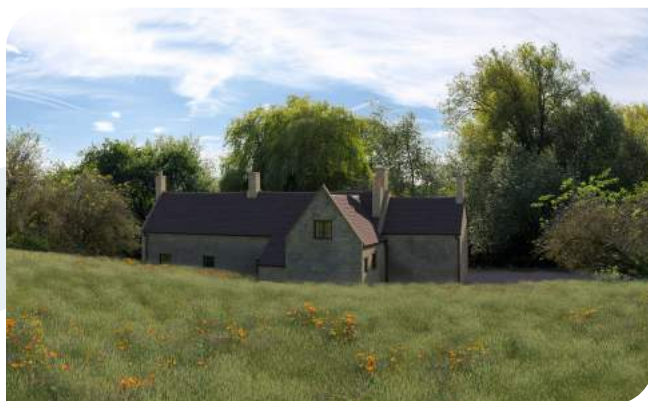
Photomontage showing how Cooks Hole Farmhouse could look once restored. The restoration materials for the building will be agreed with the Conservation Officer at the time.
