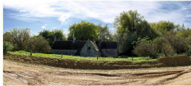
Existing view of Cooks Hole Farmhouse looking south.
