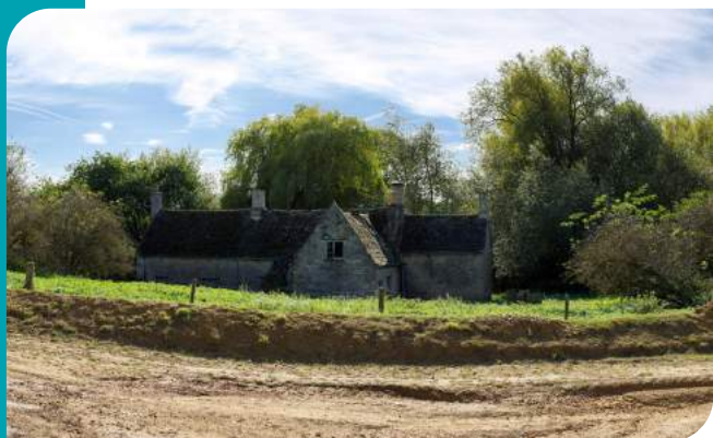
Existing view of Cooks Hole Farmhouse looking south.
